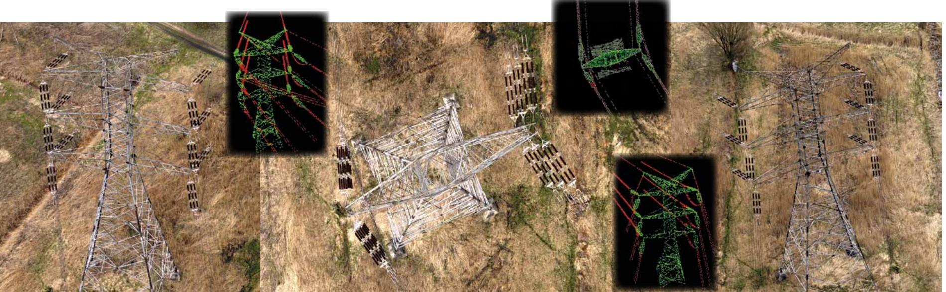
Example of a Powerline Survey - 2 DigiCAMs Oblique, 1 DigiCAM Nadir with LiteMapper , LiDAR Laser Scanner System
